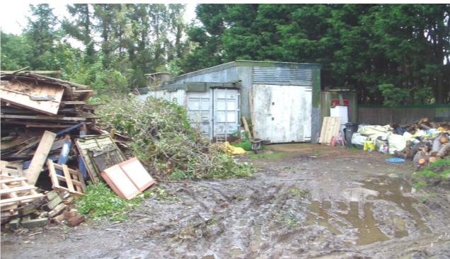
Old Structure, Concrete Base, Established Use. No Planning needed, Could be Rebuilt As A Fishing Lodge
