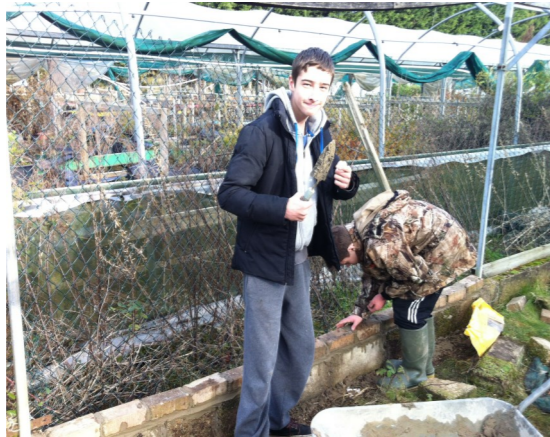
Very Basic Bricklaying Skills Being Learned As They Construct The New Chicken Run!
