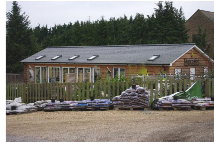
Newly Built Offices, ideal for Relocation Of Our Portsmouth Office
