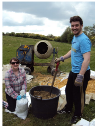
Bridge Builders In Action
